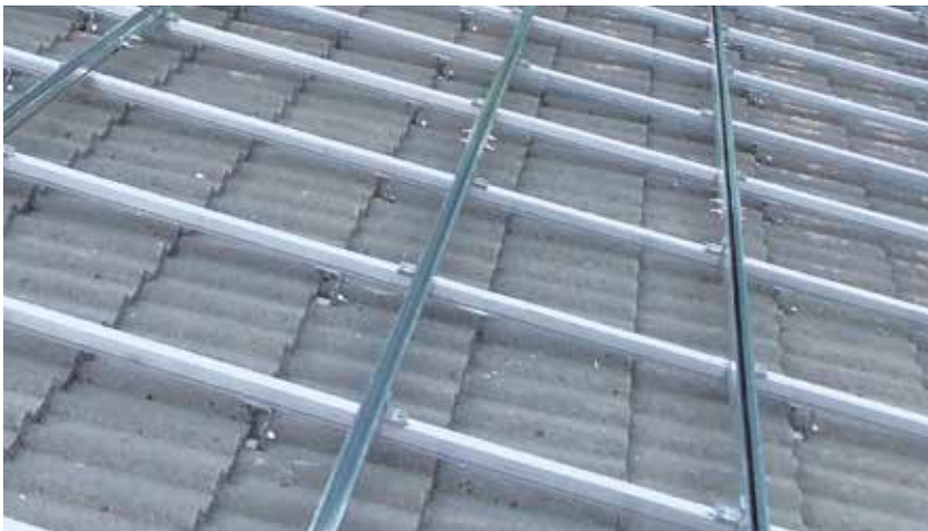
Elpo | Pfunders - Italy System: 484,65 kW | Vario 2 roof fastener with cross bracing
