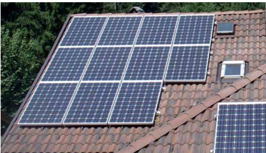
Elpo | Ehrenburg - Italy System: 5,04 kW | Roof fastener system
